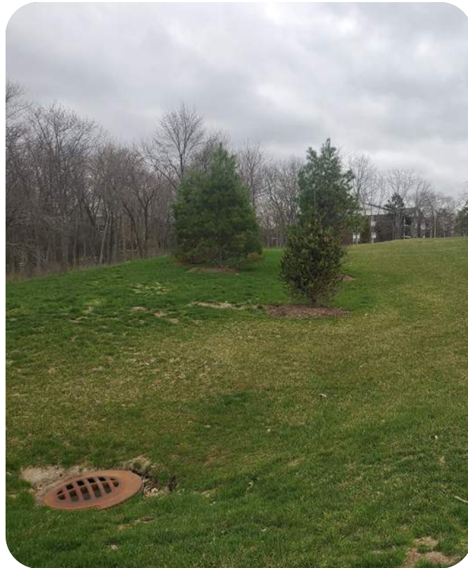
Several inlets on site fail to capture water as it travels from the eastern side of the site down to Crooked Lake.
