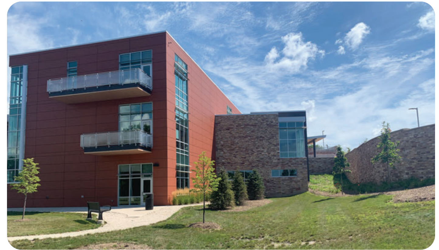
Existing entry from the building to the outdoor space.
