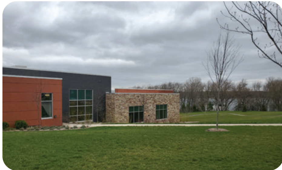
While the library has several entry points, access to most of these doors is restricted to fire egress only.
