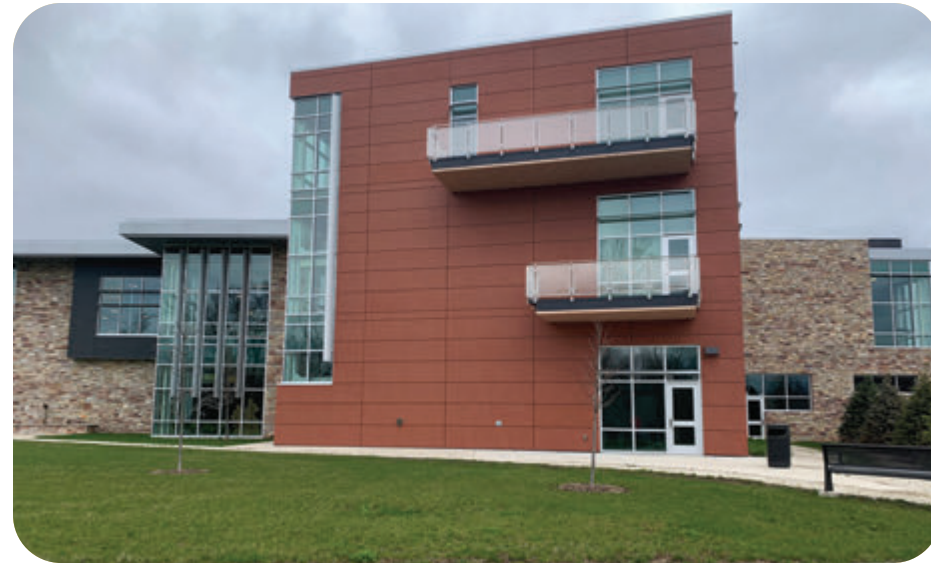
Balconies provide elevated views to Crooked Lake and the woodland around the library.
