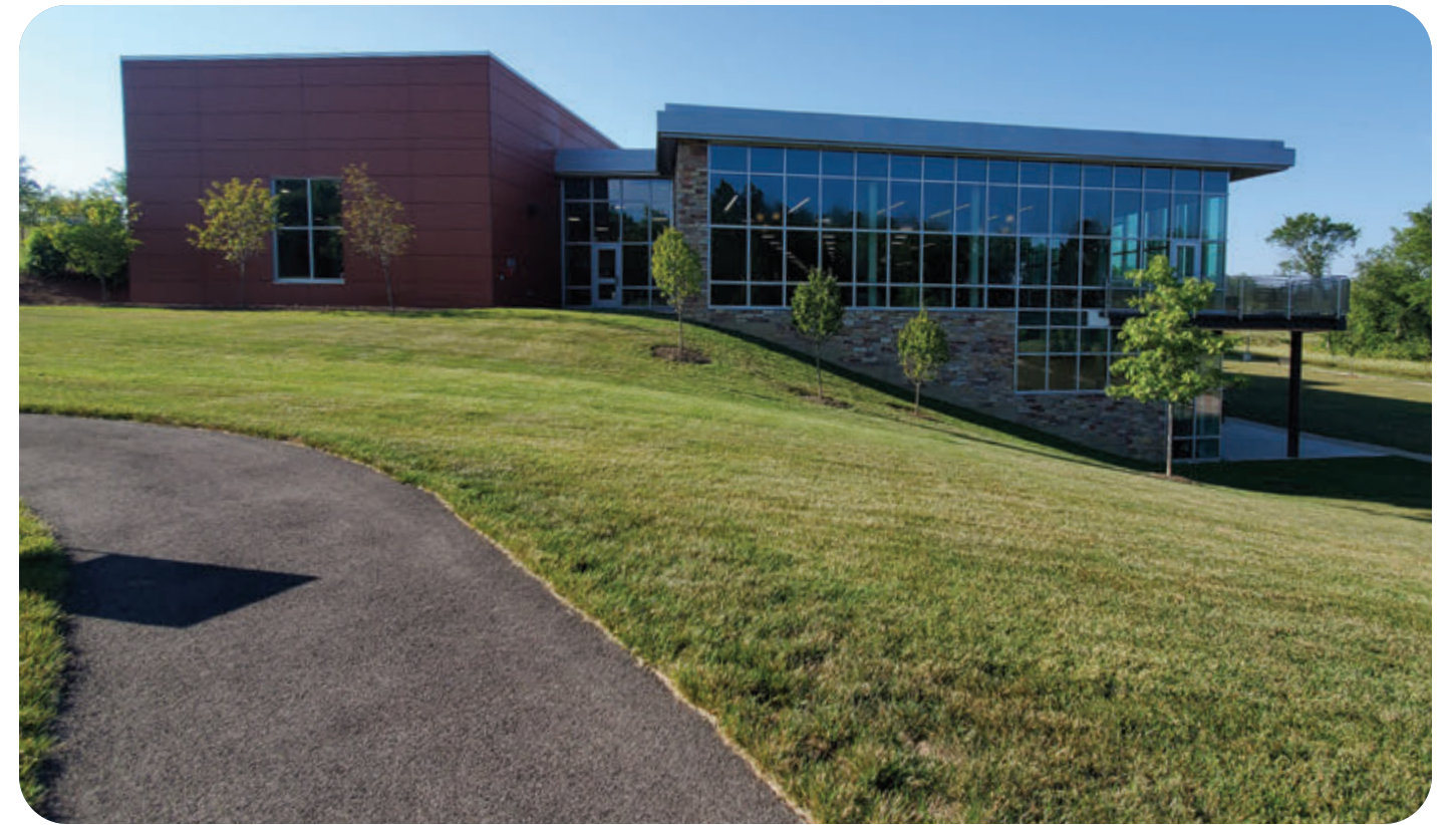
Existing slope from the east parking lot and north door to the Great Lawn area.
