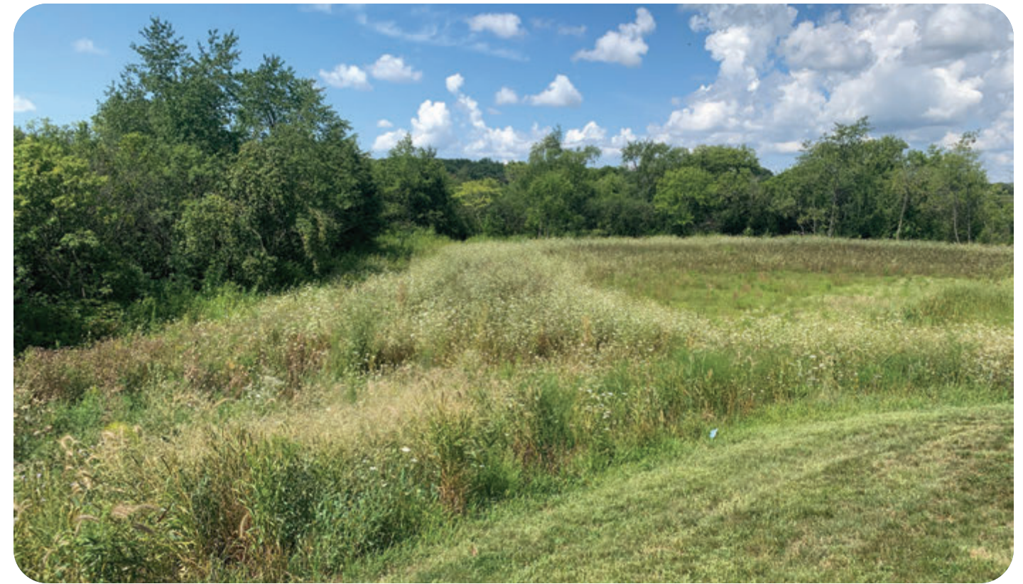
Existing condition of the stormwater basin, showing clogged underdrain.
