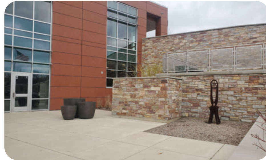
Existing sculpture begins to create a quiet space & focal point but still lacks furniture and planting to support the space.
