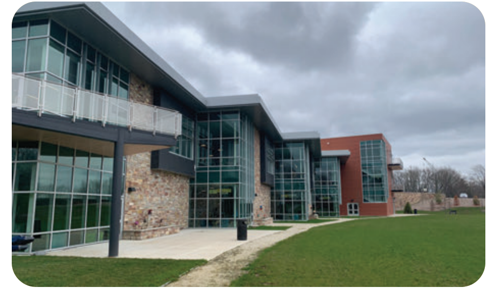
View looking south of the library showing open window views to the surrounding natural areas.
