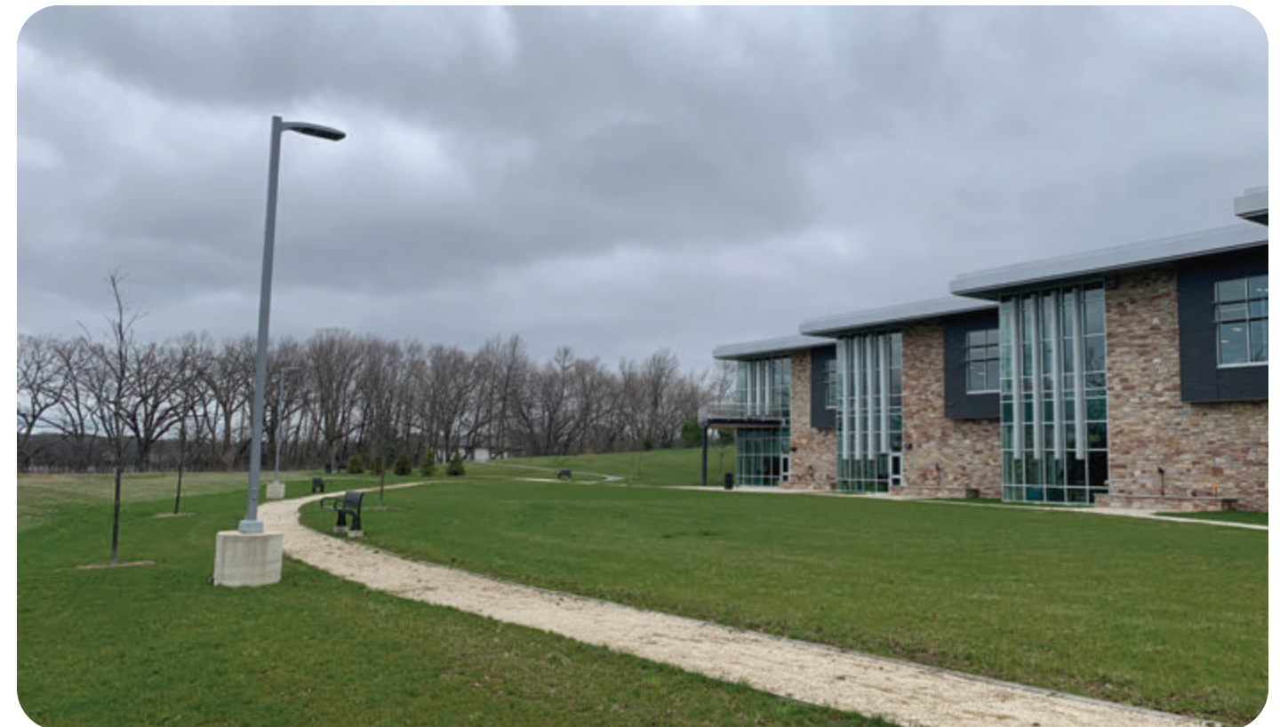
Light fixtures are located around the existing main loop. Light features should be kept at a minimum to discourage after hour visitors.
