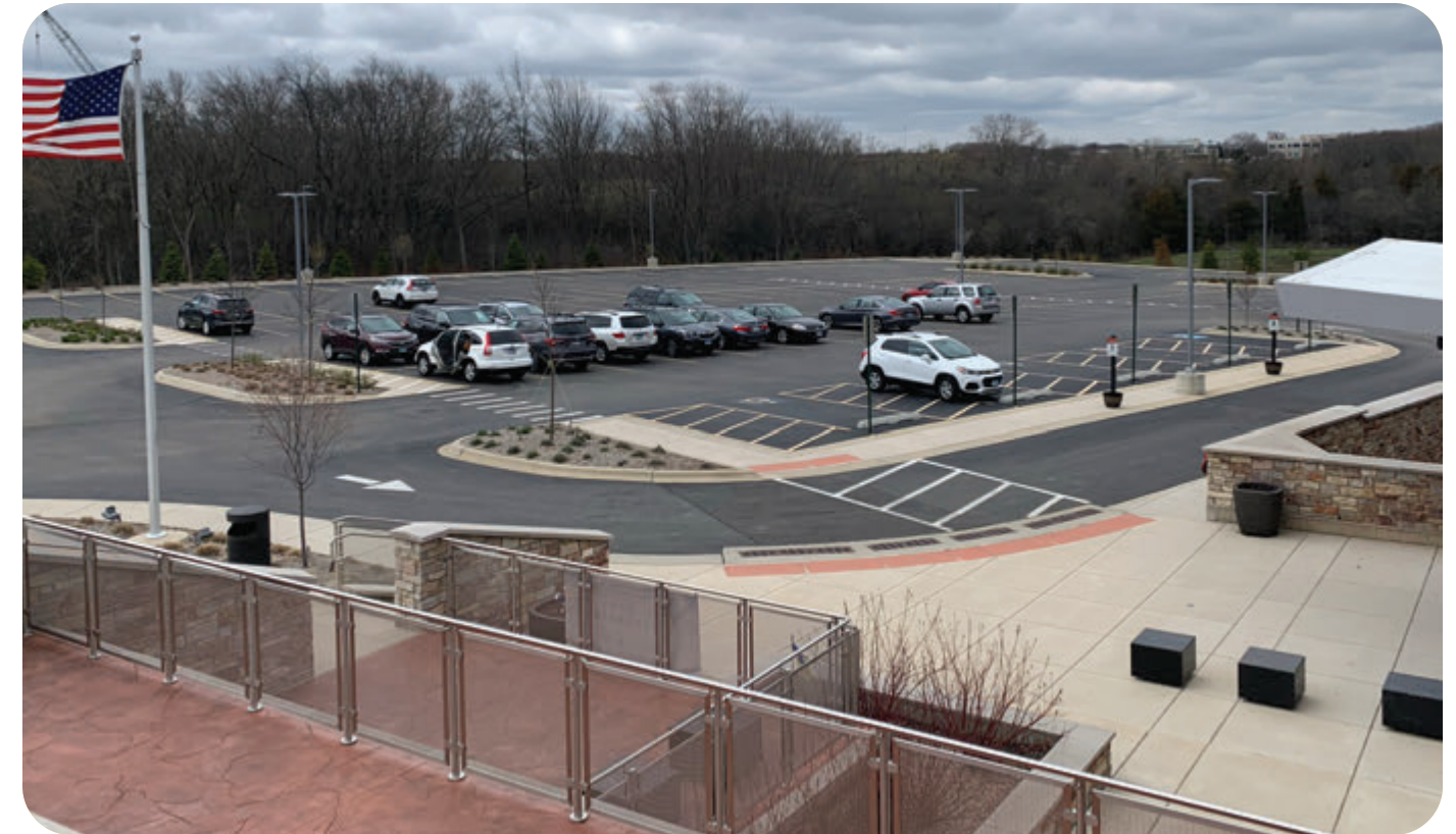
View of the south parking lot with the woodland tree canopy in the background. The south parking lot provides access to the main entrance.
