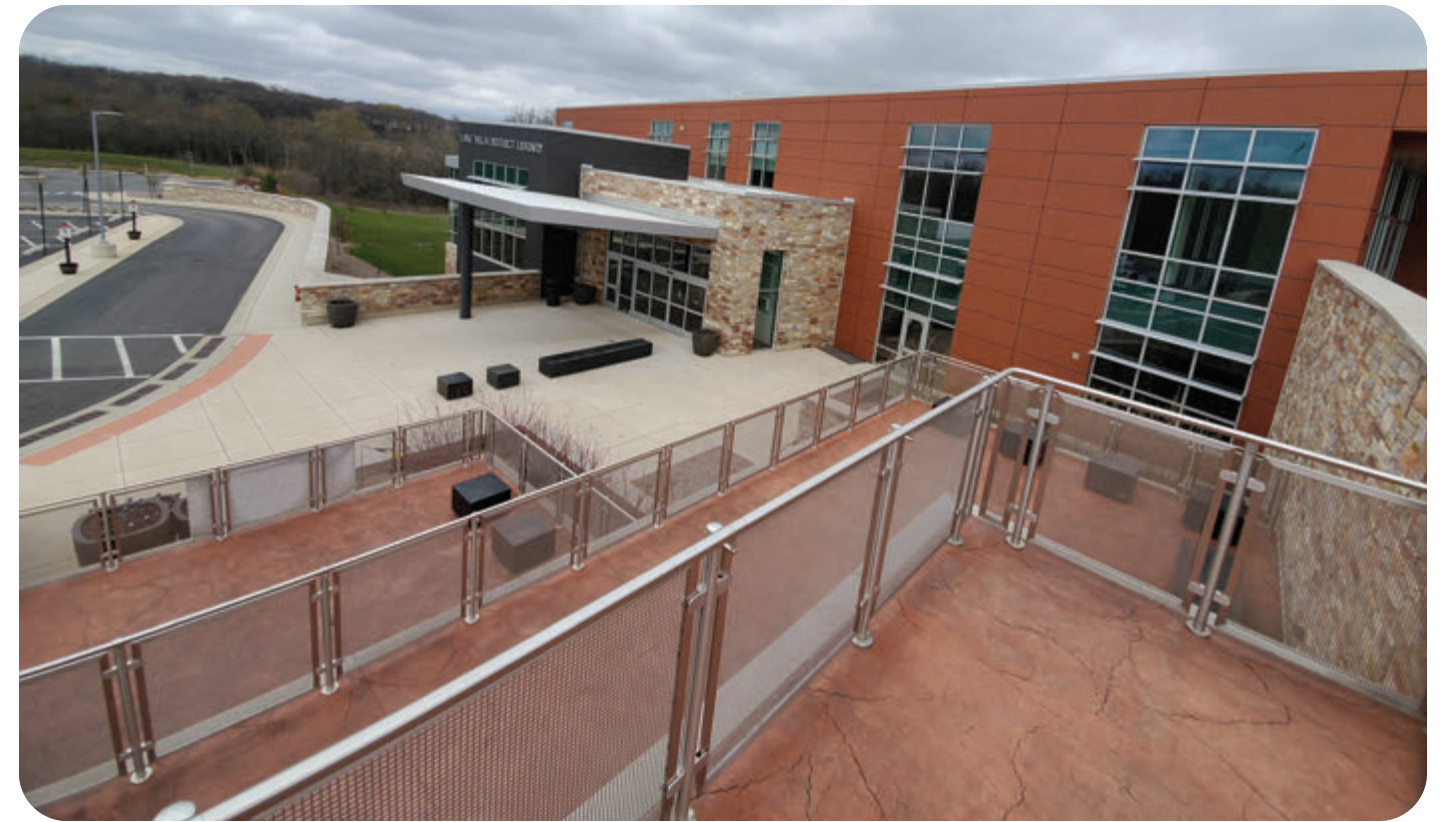
The existing terraces located southeast of the library lack relief from the bright sun.
