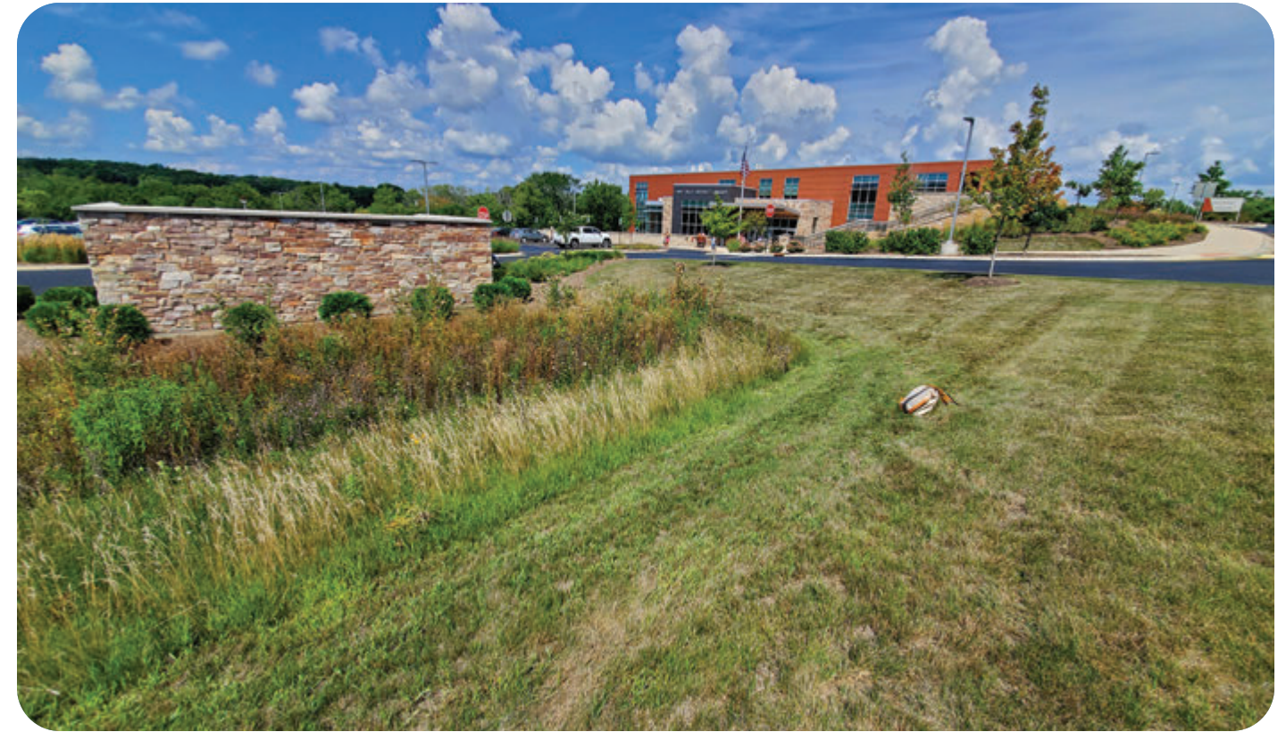
Existing rain garden on the eastern side of the south parking lot.
