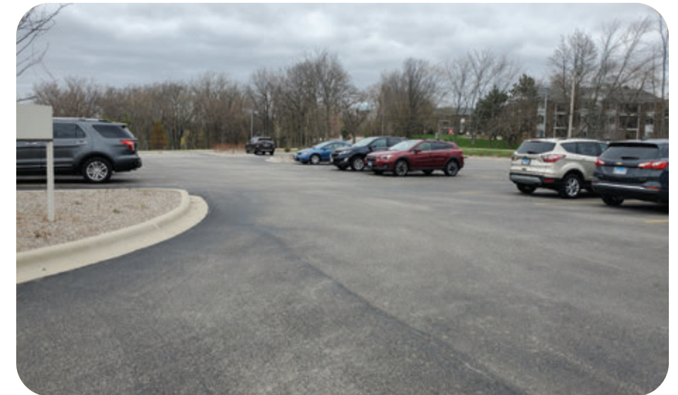
The east parking lot includes a geothermal heating system.
